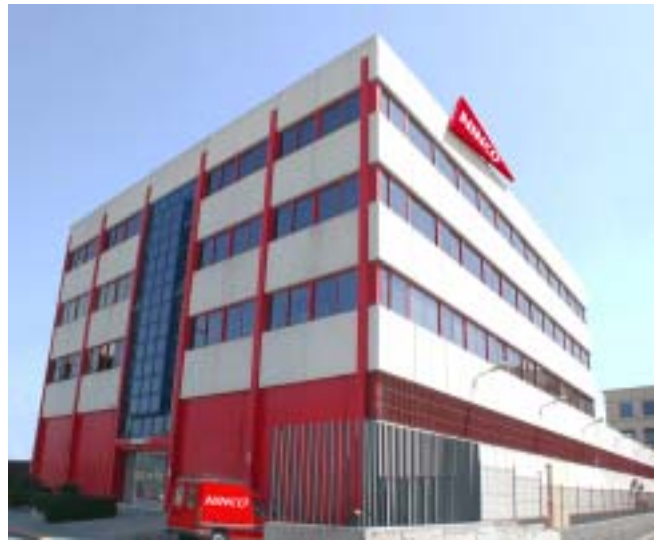
The impressive Ninco building
